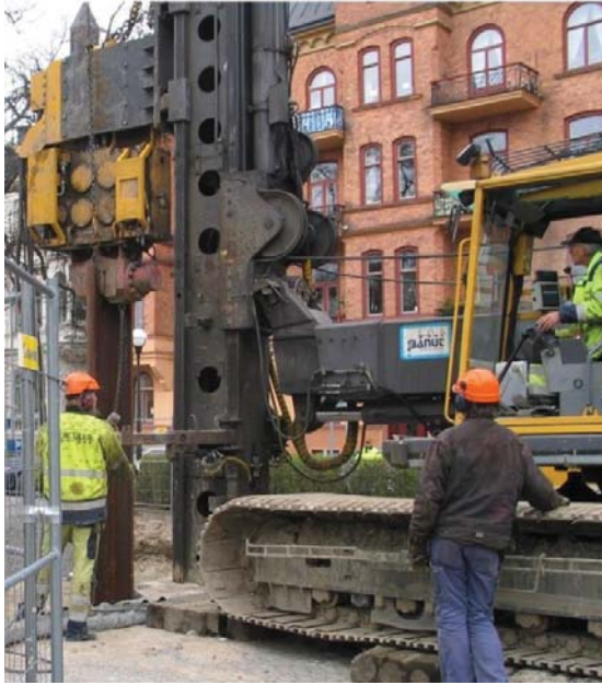
Figure 3.4 Photo of driving equipment used in the Karlstad theatre field test.
